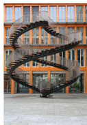
Photo of Endless stairway at KPMG, Munich, Germany by Oliver Raupach. Creative Commons Attribution-Share Alike 2.5 Generic
